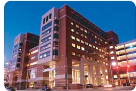
UAB Hospital, located on the University of Alabama at Birmingham campus
